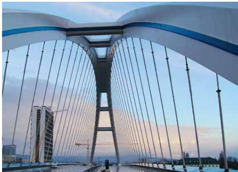
Photo made few weeks after the bridge has been rotated (bridge still doesn't have the pavement and the protectors of the hangers are not installed).
