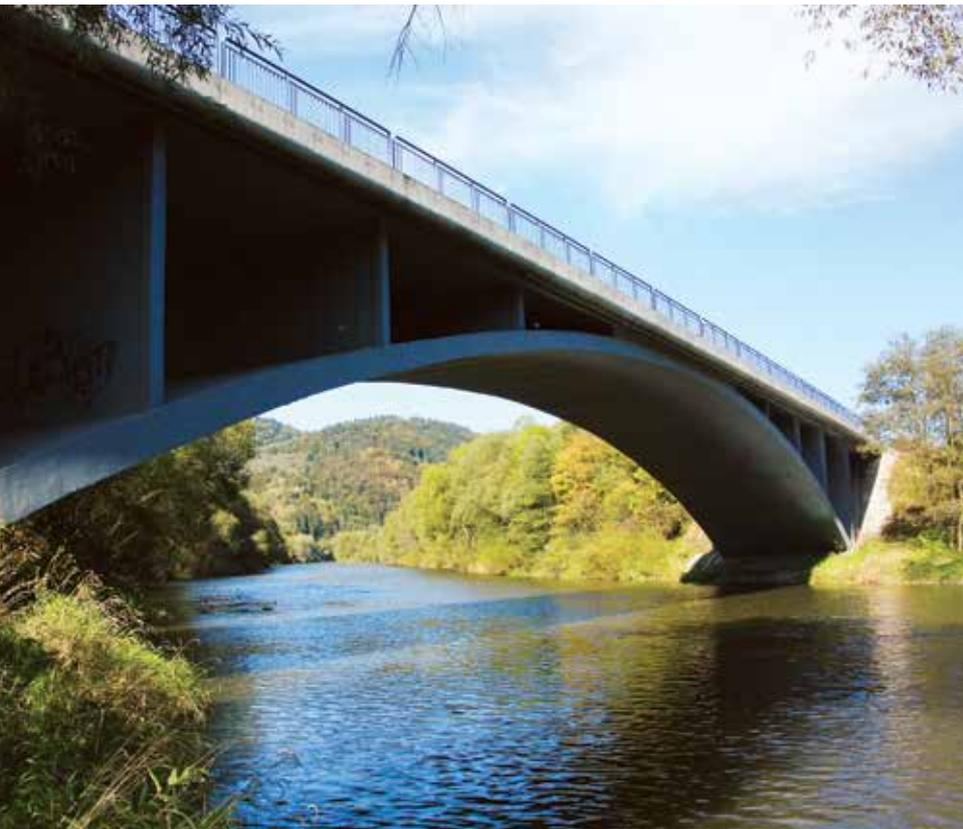
In the year 1924 an approximately 64 m long reinforced concrete bridge was built near the village Dlhá nad Oravou, which is also referred to as the bridge of Masaryk.
