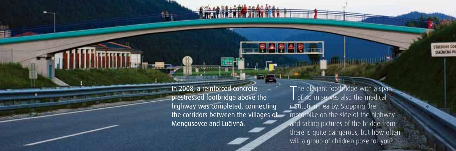
In 2008, a reinforced concrete prestressed footbridge above the highway was completed, connecting the corridors between the villages of Mengusovce and Lučivná.
