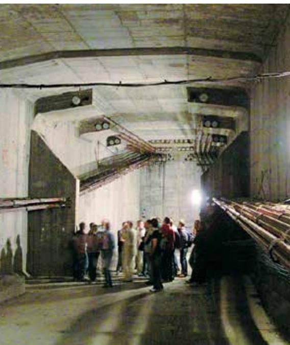
The inside view of the bridge chamber (above the pier, the chamber is 8.5 meters high)
