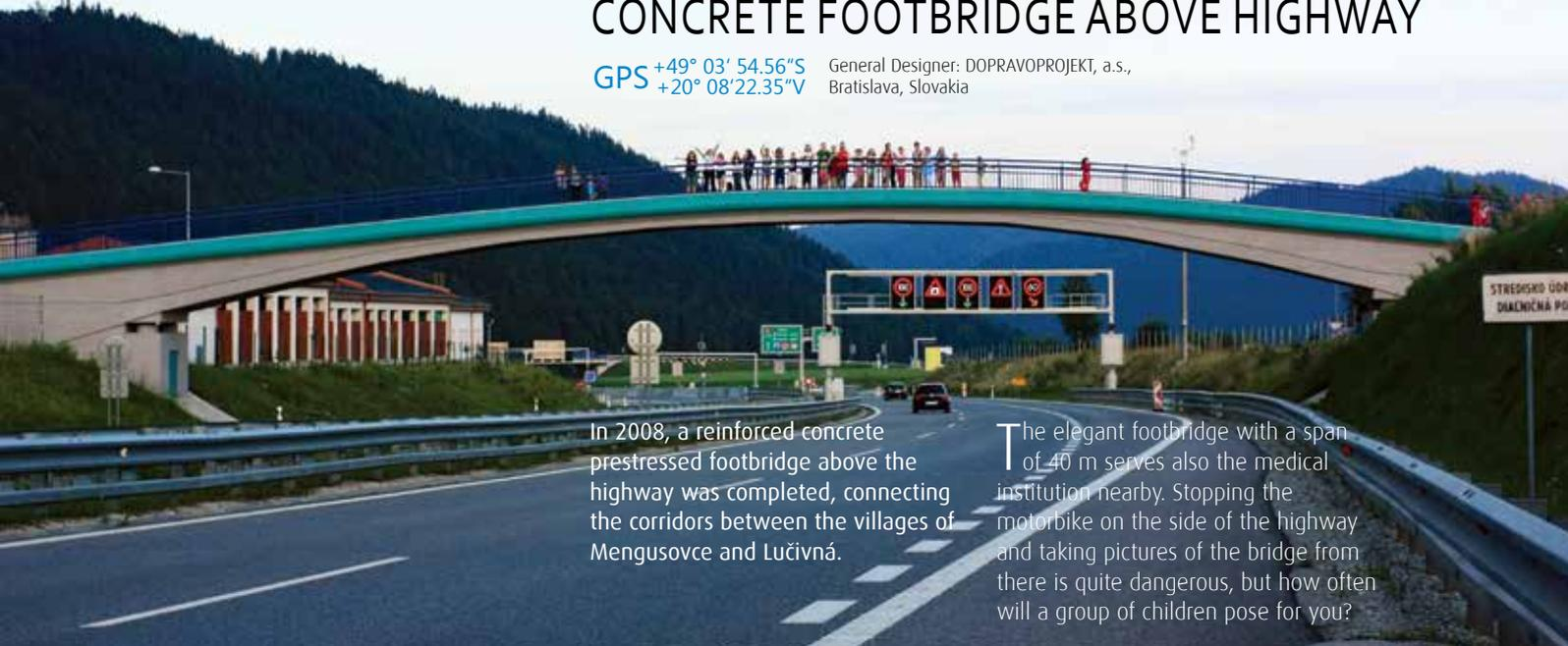
In 2008, a reinforced concrete prestressed footbridge above the highway was completed, connecting the corridors between the villages of Mengusovce and Lučivná.
