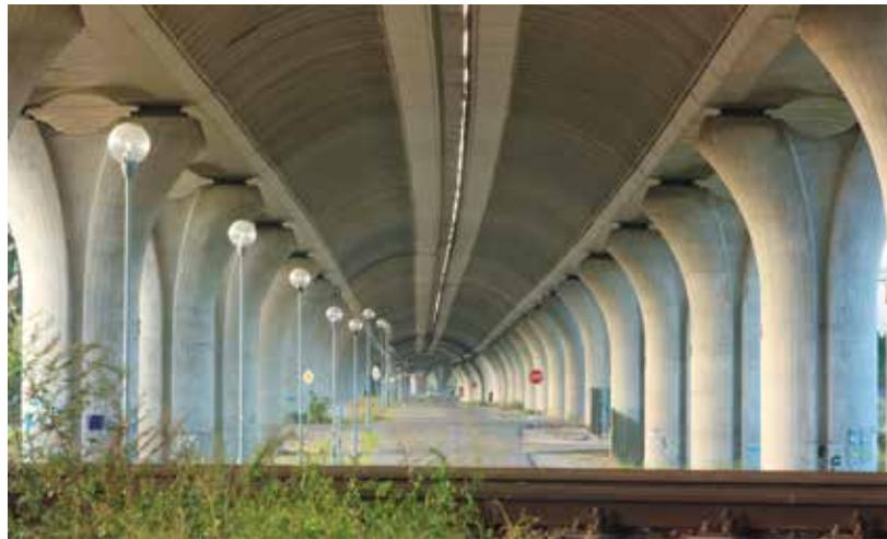
of this, the 139 piers and the shape of the superstructure had careful attention. A non-standard solution of the structure is achieved mainly by the unconventionally shaped struts supporting the upper slab of the box girder, which, together with the piers, forms an interesting appearance.
