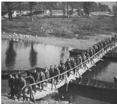
Small towns, where rich social life flourished after the working day, needed temporary bridges leading to the working site to be built for them. The construction was significantly complicated in 1952 with the discovery of a mineral spring, which has been ever since used in the nearby Spa Nimnica. As a matter of fact, the effect of a mineral spring on concrete is opposite to the effect on a human
