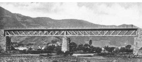
Near Margecany, over the river Hornád on the railway between Červená Skala and Margecany, there was a truss bridge which was later moved few meters downstream using some of the supports of the old bridge. Today, none of them exist anymore, but their abutments and a part of the piers are still visible. Abutments were later used as a supports for the pipeline bridge.
