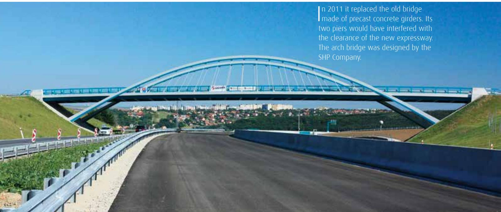
In 2011 it replaced the old bridge made of precast concrete girders. Its two piers would have interfered with the clearance of the new expressway. The arch bridge was designed by the SHP Company.
