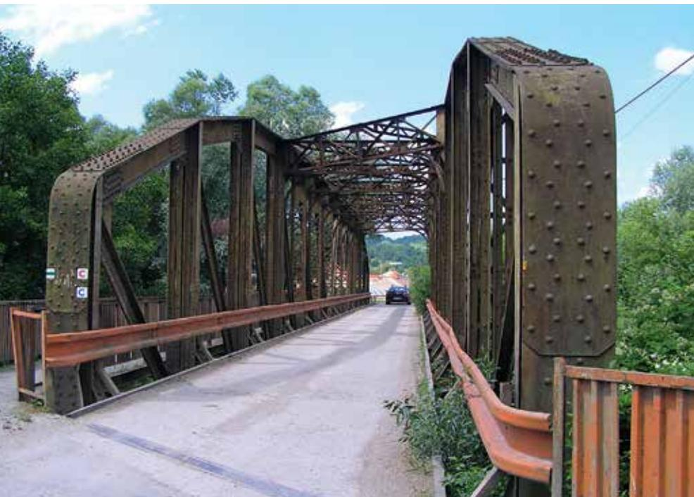
The road bridge across the river Hron with a span of 57 m was originally a railway bridge and it was transported to its contemporary place when the railway administration put it out of service.
