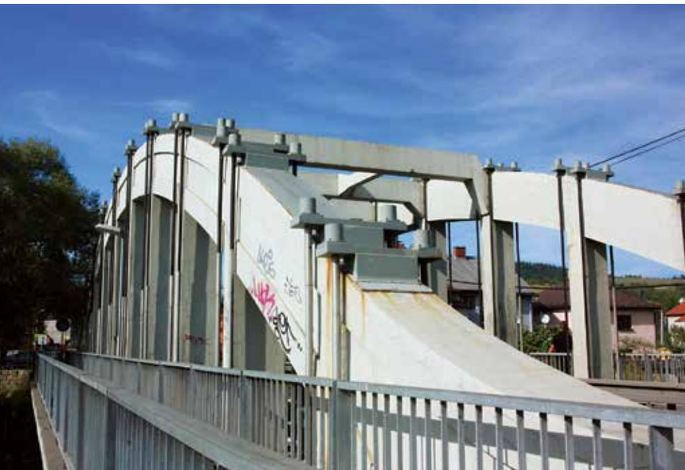
Nearby the border crossing with the Czech Republic, a concrete bowstring arch bridge with a span of 32 m crosses the river Čierňanka. The reinforced concrete bridge was built in 1931, but due to its poor technical state, it had to be strengthened in 2002 by massive steel profiles anchored to the arch of the bridge.
