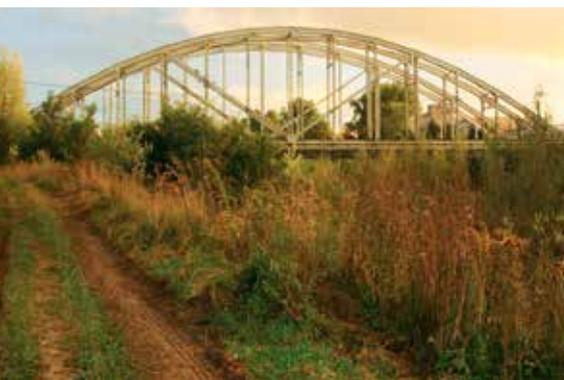
The first railway bridges were built here within the railway line between Košice and Bohumín, which was begun to be built in 1869. The original bridge was rebuilt in 1911. It had three truss arch spans of 34.5 + 44.8 + 34.5 m. Next to it, there was a newer bridge from the year 1938. As the other bridges, these were also completely destroyed at the end of the war, without any possibility of reconstruction. Thus, a new timber temporary bridge had
