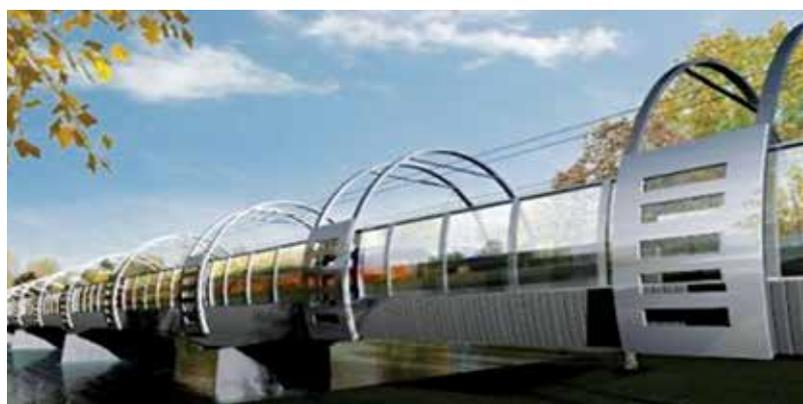
up until 1984 when a new through truss structure with parallel chords was built. Nowadays, plans for the new bridge are ready. It is to be next to the old one which afterwards will be used only by pedestrians and cyclists. The new superstructure will be made of prestressed concrete and will be 340.6 m long. The maximum span will be 52 m. The author of the project is the company Reming Consult in cooperation with the Betoning Company. The construction is already in progress.
