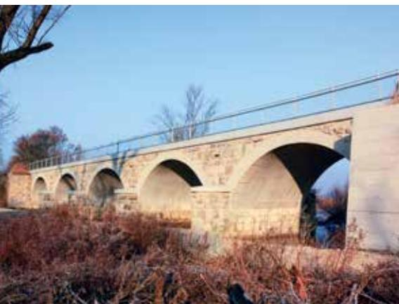
Reconstructed arches, which were originally made of stone
