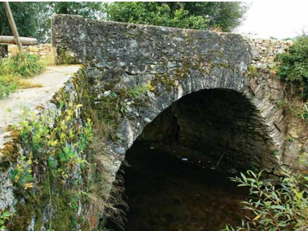
The stone arch bridge, with a clear span of approximately 7 m, situated near the village, spans the Rimavica stream.
