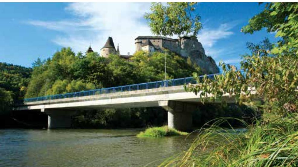
Since a long time ago, there has been a bridge under the Orava Castle crossing the river Orava. At first it had a timber structure, then its superstructure was made of steel girders and finally, from the year 1989, the 90-m-long bridge has been made of precast concrete girders.
