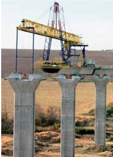
In this technology, the segments are progressively connected to the already finished structure. Construction can proceed by balanced cantilevers or by a system of one-sided cantilevers with sufficient stabilising of the structure during its construction by means of stays or temporary supports. In the case of a concrete bridge, special falsework is mostly used, the so called overhead launching gantry, which is able to move on the finished part of the structure. The launching gantry is equipped
