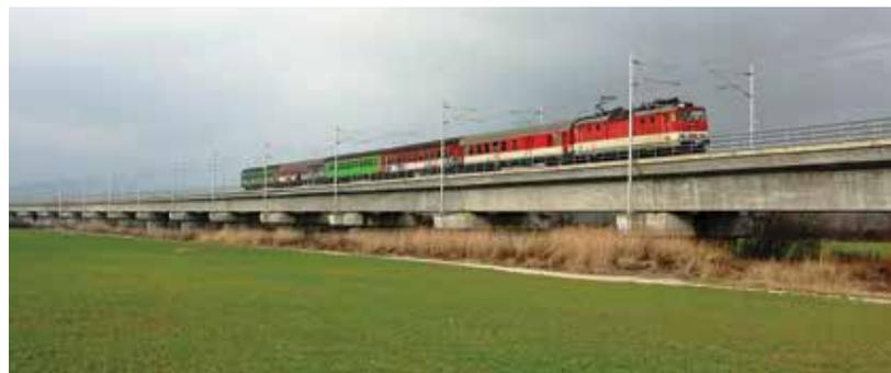
Designers proposed a bridge instead of high embankments concerning its possible excessive settlements caused by weak subsoil conditions. After several proposals of different types of steel bridge in the final
