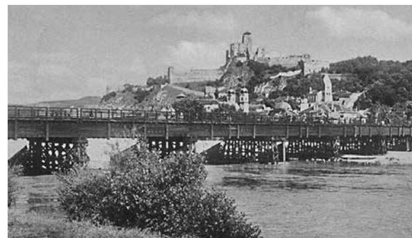
The temporary timber bridge after the destruction of the original bridge in 1945
