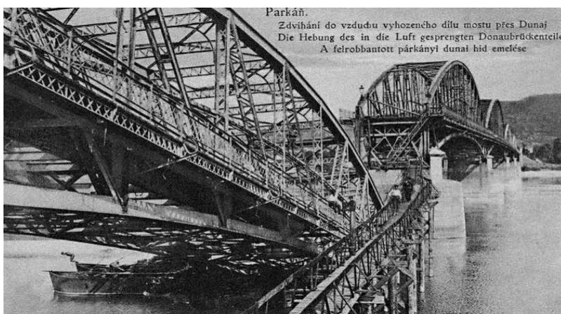
Temporary footbridge and the preparation works for the reconstruction, 1922
