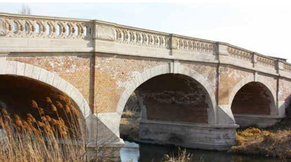
Italian constructors and stonemasons built it following the design of MSc Ján Nagymihály from the year 1903. This 42 m long bridge has a stone arch made of limestone completed by red bricks on the sides. Its three arches have clear spans of approximately 5 m. The bridge was reconstructed in the year 2007 and on this occasion a commemorative stamp was issued.
