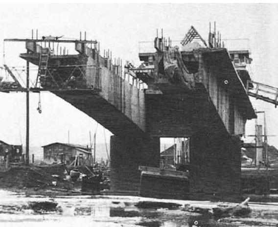
The free cantilevering method is presently used to construct segmental bridges with medium spans between 50 and 80 m.
