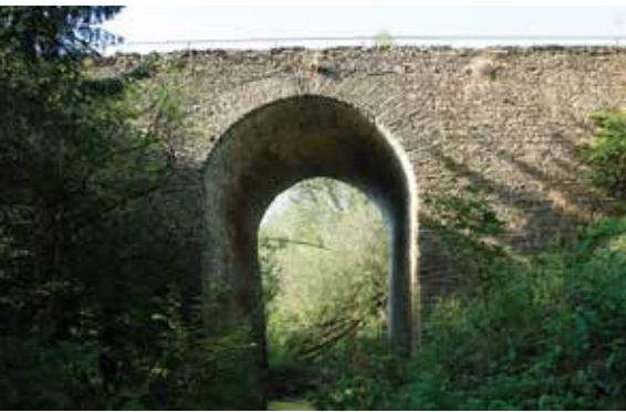
The bridge crosses a small valley of a stream at a height of approximately 10 m, with the clear span of the arch being 5.8 m long and 9.4 m high.
